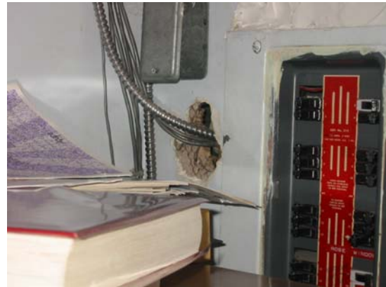
Figure 17: Hole in Wall
